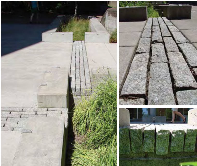
Cobble stormwater conveyance trenches are created by embedding spaced cobbles in a concrete trench. Small gaps between the stones allow water to move through the trench.
