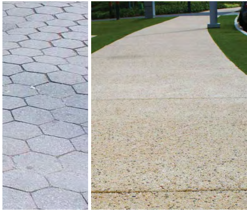
Asphalt Hexagonal pavers (left) and exposed aggregate concrete (right) help the park fit into the larger context of the Schuylkill river park and the larger Philadelphia park system.
