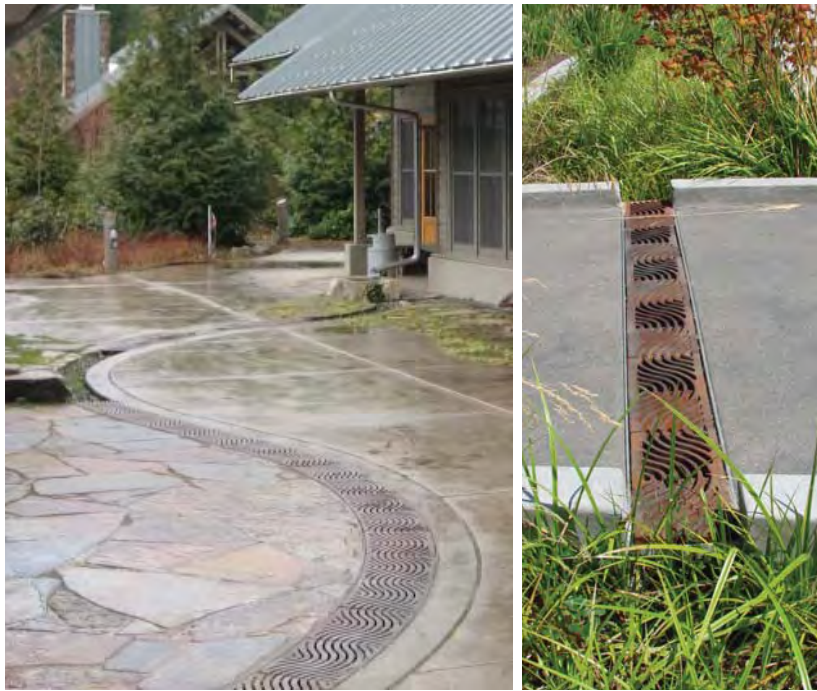
Trench drains with decorative iron grates can move large quantities of stormwater in a visible way.
